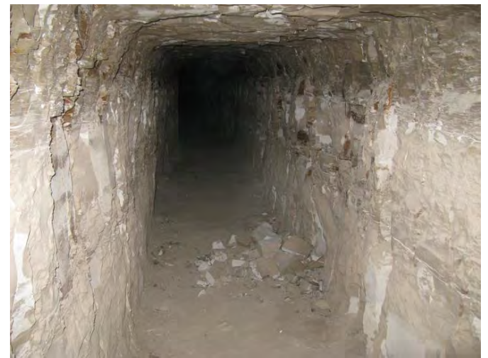
Tunnel leading to the man chamber
